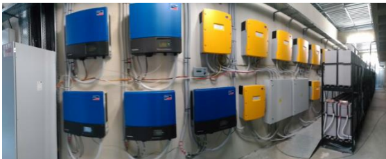
Figure 3: The inverters and the batteries of the autonomous microgrid of the AUA library
