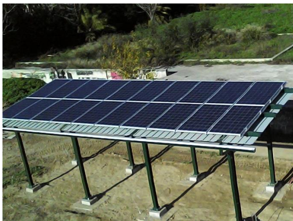
Figure 7: The PV shelter
