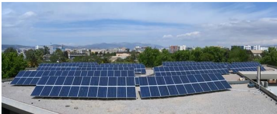
Figure 2: The PV installation in the library's roof
